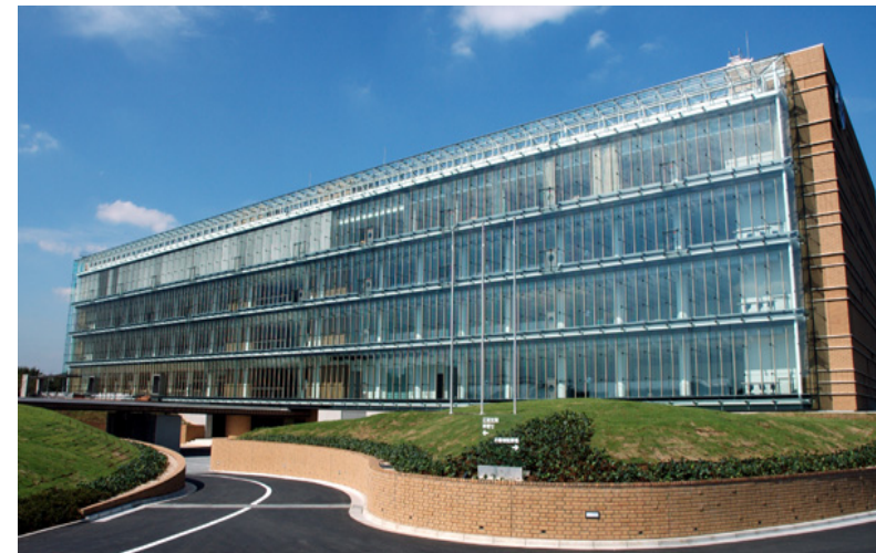
Mabuchi Motor's Matsudo Head Office building which was awarded the Sustainable Architecture Prize
