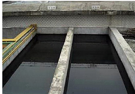
Settling tank for recycling wastewater
